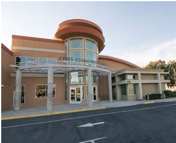
Photo 11 - Ceres Community Center
