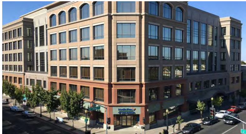
Photo 1- Tenth Street Place
