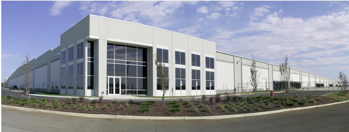
Clean lines, articulated structural bays, and different materials can be used to break up the mass of large buildings.
