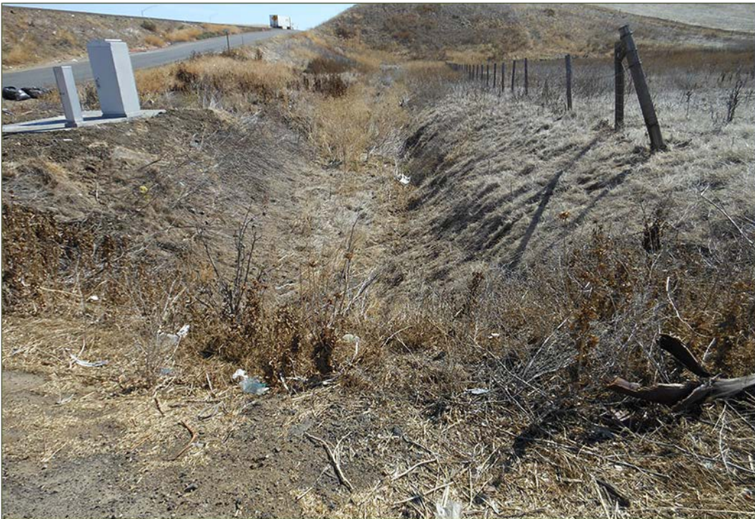
Roadside ditch (Dx) along southbound ramp onto I-5.
