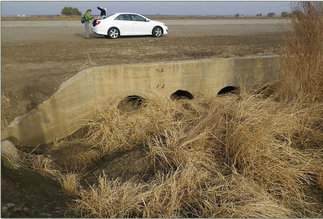
Little Salado Creek is culverted under the runway.
