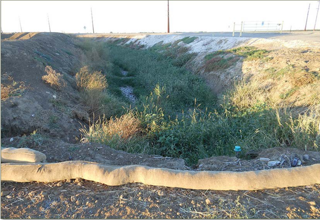
Agricultural ditch (D8) crossing Marshall Road parallel to Delta-Mendota Canal (sample point 4).
