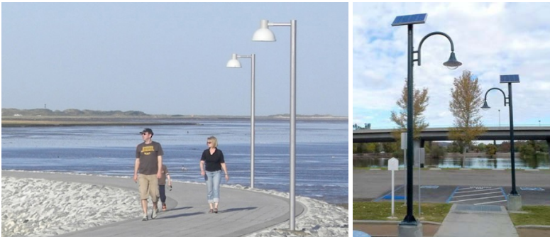
Examples of pedestrian scaled lighting, including solar powered fixtures
