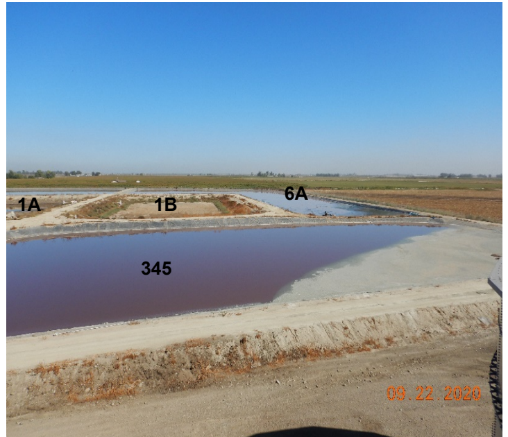
Photo No. 14: Looking northeast from a bioreactor treatment tank at the wastewater ponds.
