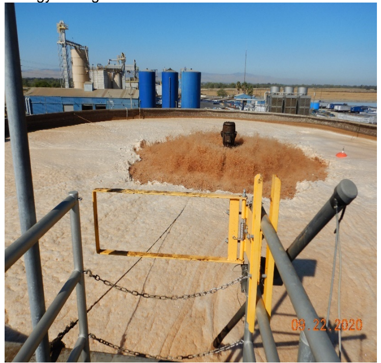
Photo No. 12: Aerator operating in one of the of the bioreactor treatment tanks.
