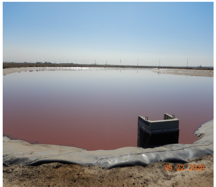
Photo No. 20: Looking east at wastewater pond 6A which is HDPE lined.
