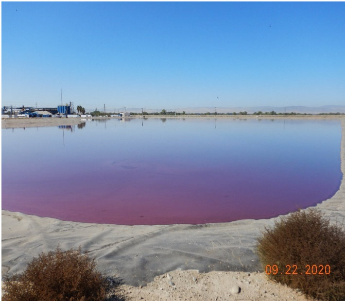
Photo No. 21: Looking west at wastewater pond 6B which is lined.
