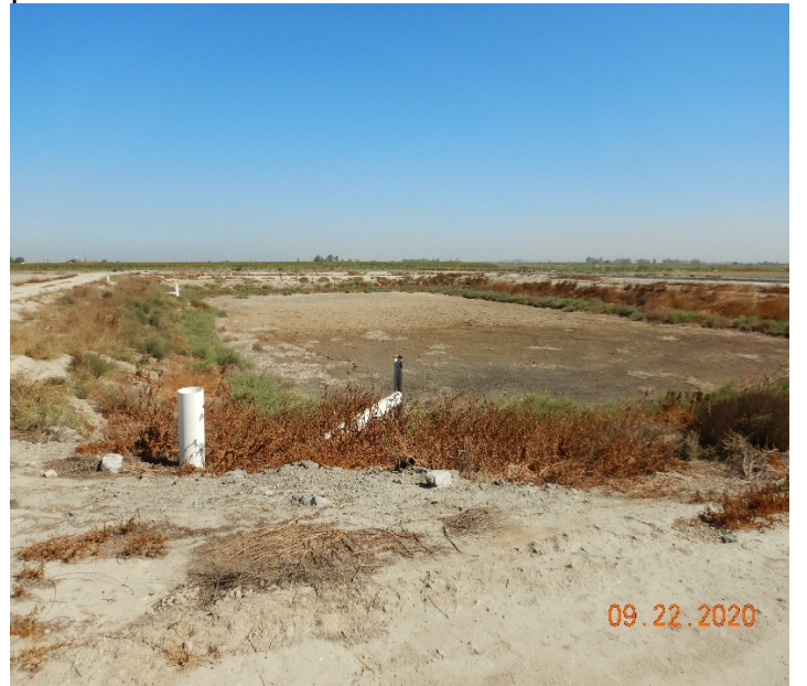
Photo No. 16: Looking north at Wastewater Pond 1B.
