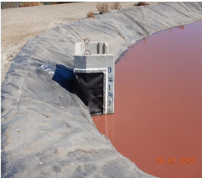
Photo No. 19: Freeboard markings on flow structure in one of the HDPE lined ponds.
