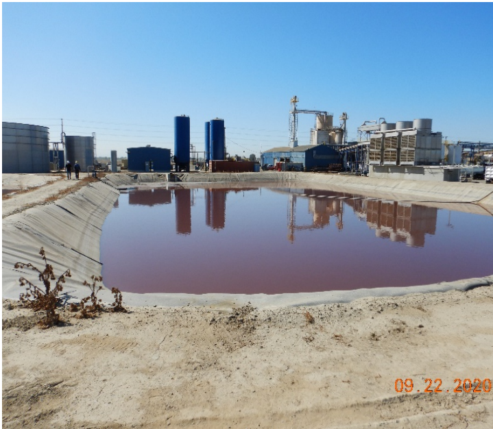
Photo No. 17: Looking north at Pond 2 which is HDPE lined.
