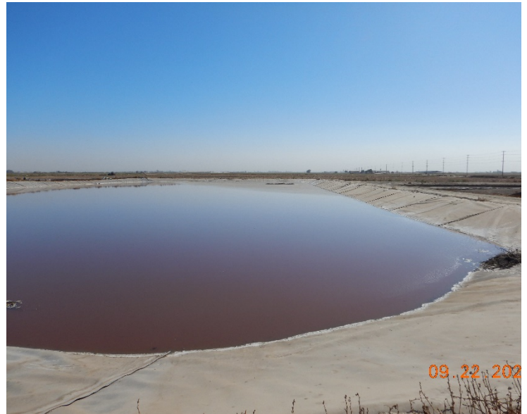
Photo No. 18: Looking east at Pond 345 which is HDPE lined.
