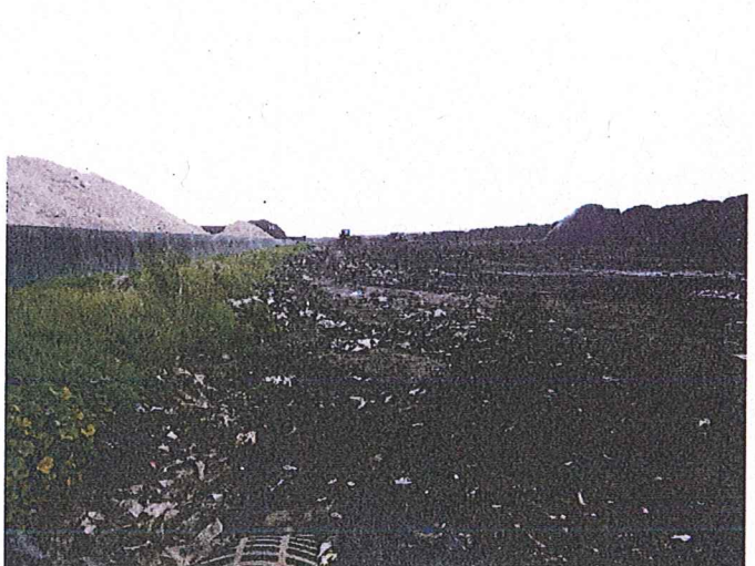
Figure 12 Standing in the same location as Figure 11, but looking southeast/downstream along the eastern leachate control berm and a drain that flows to the East Pond.
