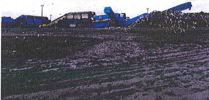
Figure 33 Raw Compost Receiving and Processing Area. The ponding in the foreground is atop a yet to be finished composting pad.
