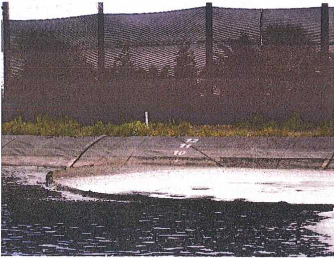
Figure 7 Looking east at the East Pond's freeboard marker. Over 4 feet of freeboard was available.
