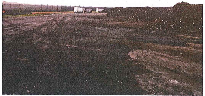
Figure 26 Composting windrows atop the finished Phase 2 composting pad.
