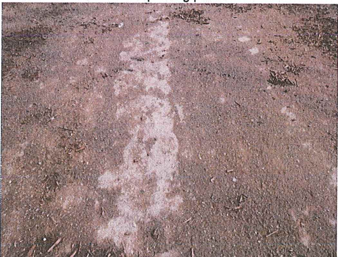
Figure 29 A close-up view of the finished Phase 2 composting pad.
