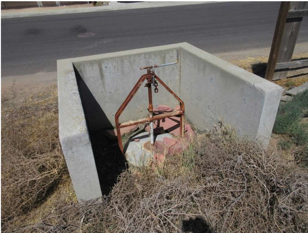
Photo 10: View of a representative irrigation system capture box located in the western portion of the subject site.
