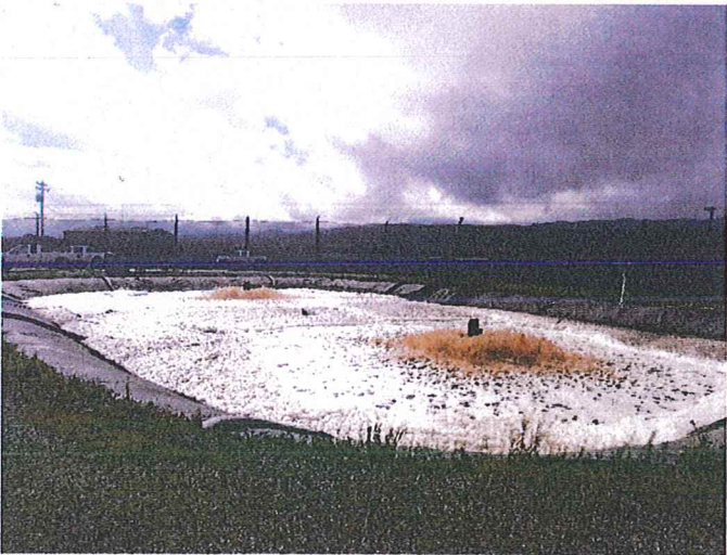
Figure 9 Looking south across the Treatment Pond. Only two of the Treatment Ponds three aerators were operating.
