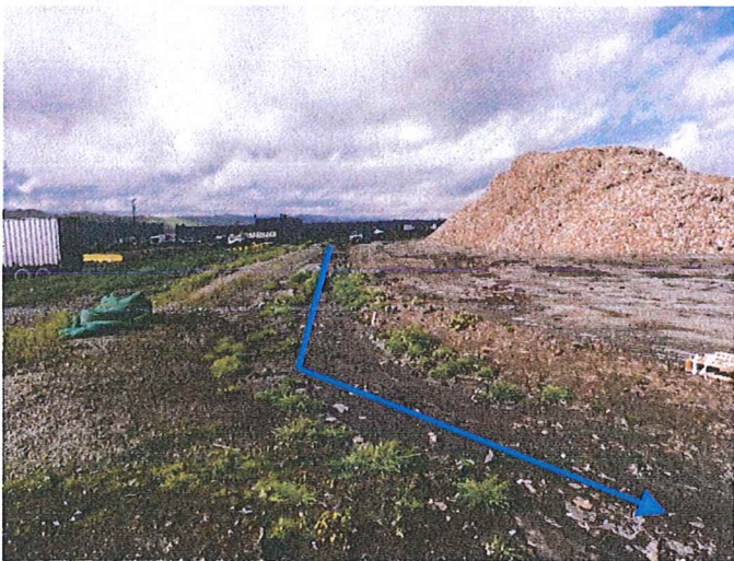
Figure 21 Looking west along the western leachate drainage channel, the blue arrow shows the leachate flow path.
