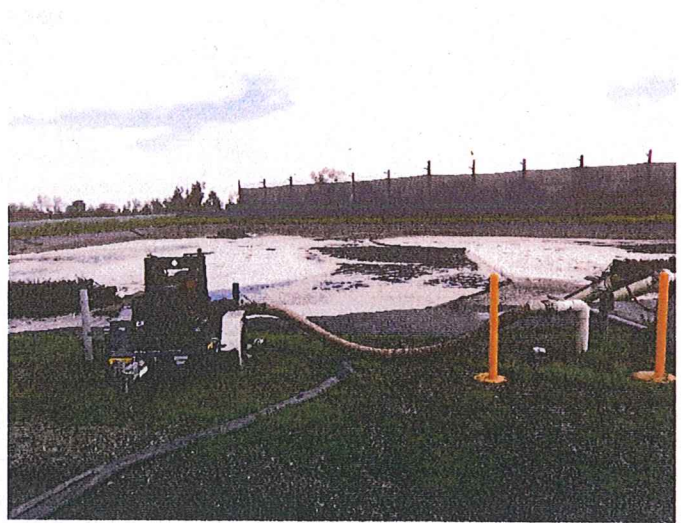
Figure 8 Looking at an additional pump along the East Pond. This pump is used to supplement existing pumps to transfer leachate to the West Pond.
