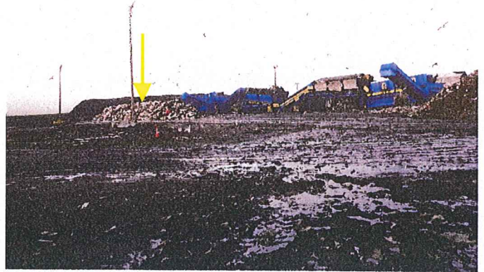
Figure 32 Raw product (yellow arrow) in the Raw Compost Receiving and Processing Area. The ponding in the foreground is atop a yet to be finished composting pad.
