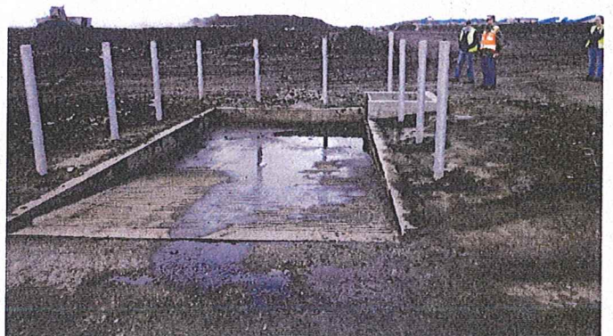
Figure 30 Looking northwest into a Catch Basin D along the central drain, that is located between the finished Phase 2 and 3 composting pads.
