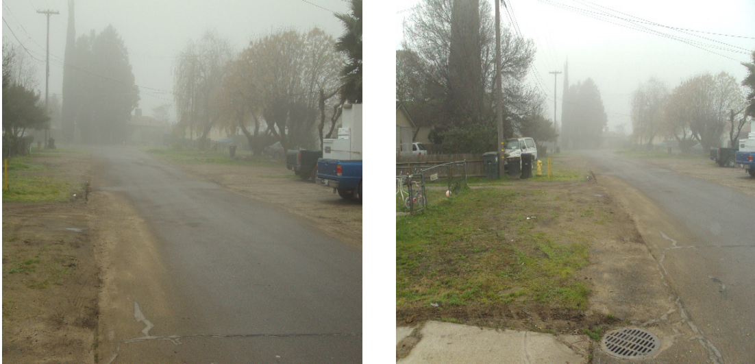
Photos reflect the need for infrastructure improvements such as curb, gutter, storm drain and ADA curb cuts along 4 th Street.
