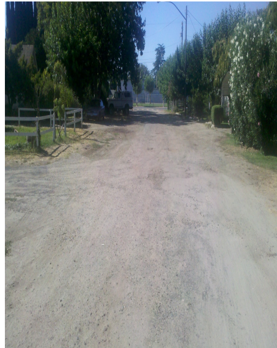
Photos reflect Covey Street (photo on left) and C Street (photo on right), which show the subject project area in need of curb, gutter, storm drain, sidewalk, and street repaving.
