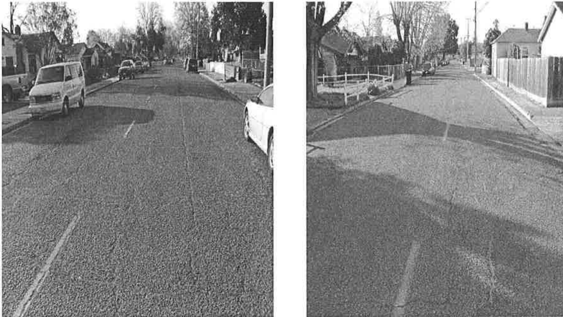
Photos reflect antiquated infrastructure in need of replacement or improvements along Davitt Avenue (Work to include underground water and sewer line replacement).
