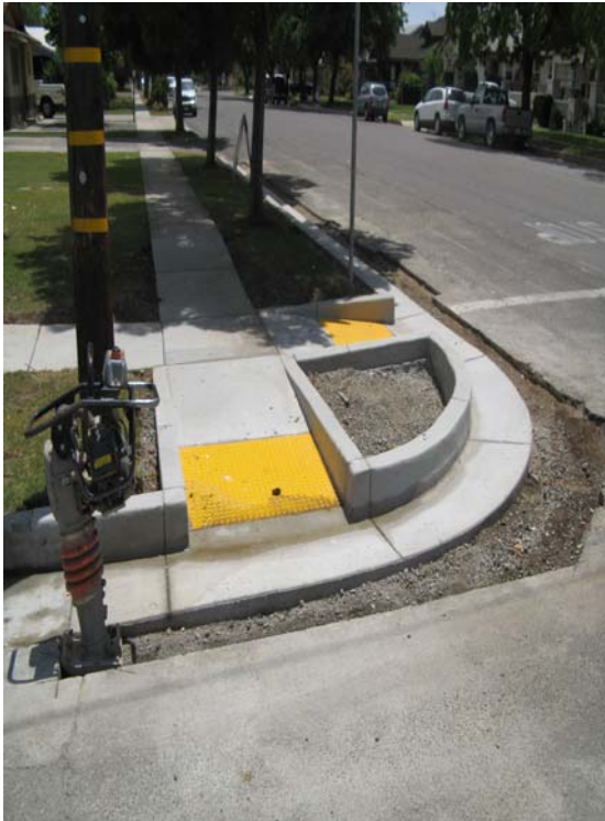
Photos reflect the installation curb, gutter, and sidewalk improvements in Newman.
