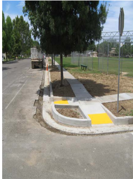
Photos reflect the installation curb, gutter, and sidewalk improvements in Newman.
