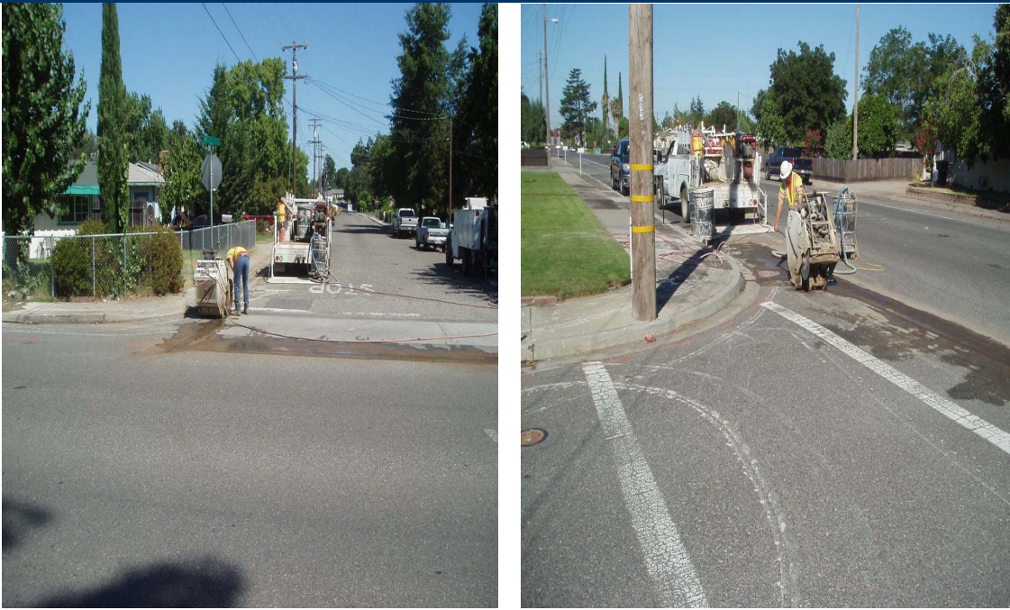
Photos reflect working crew during project construction.
