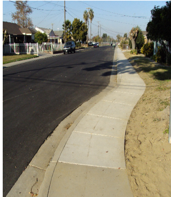
Photos reflect before and after work in downtown residential streets lacking curb, gutter, storm drain, sidewalks, and ADA ramps in Ceres.
