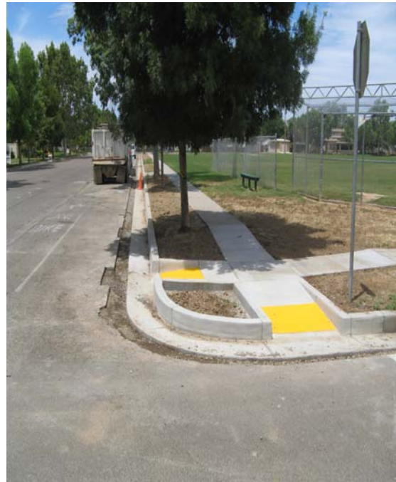
Photos reflect the installation curb, gutter, and sidewalk improvements in the project area.
