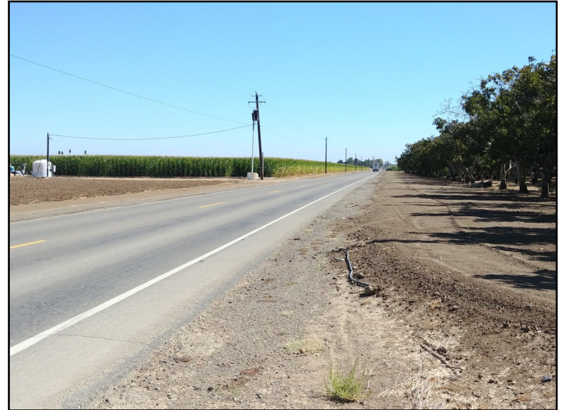
Fink Road Between Bell Road and Medlin Road, Looking East, September 24, 2019
