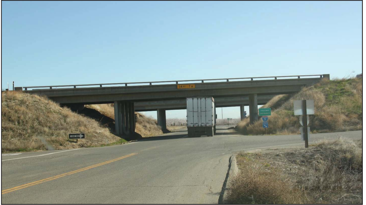
Fink Road / I-5 Interchange
