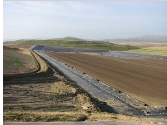
Fink Road Landfill Cell 5, Excavation and Liner
