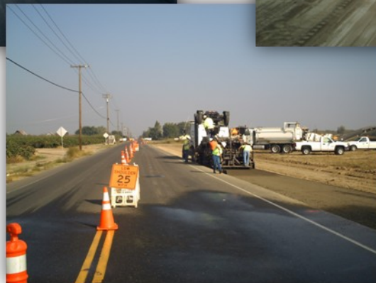
Oakdale Road Widening
