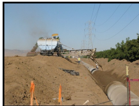
Hetch Hetchy Water Pipeline Upgrade -Western Segment
