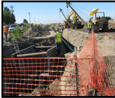
Installation of 11.6 miles of 16" diameter pipeline from Ceres to the San Joaquin River
