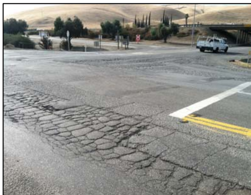
Failed asphalt on Howard Road
