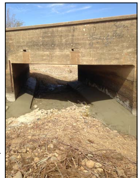
Dunton Road Bridge Scour Repair
