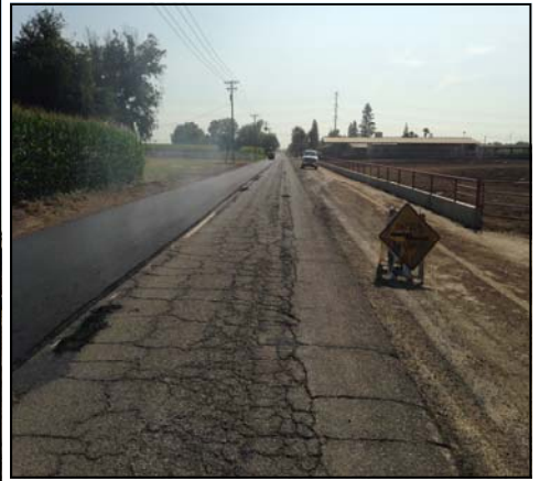
Monte Vista Avenue Paving
