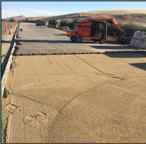
The concrete pavers were machine set by Earth Shelter Developers.
