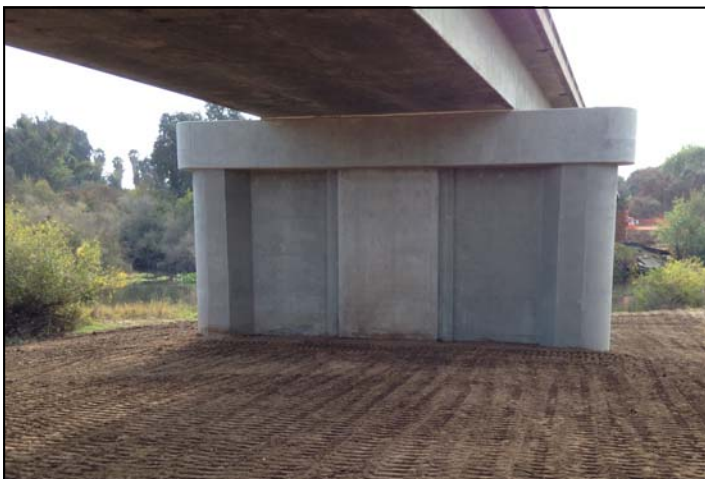
Existing Bridge Pier No. 6 after the retrofit
