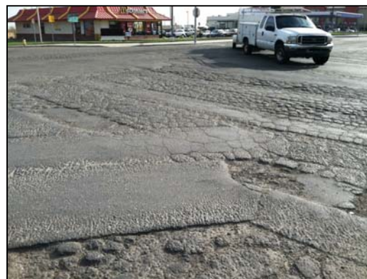
Failed asphalt on Howard Road
