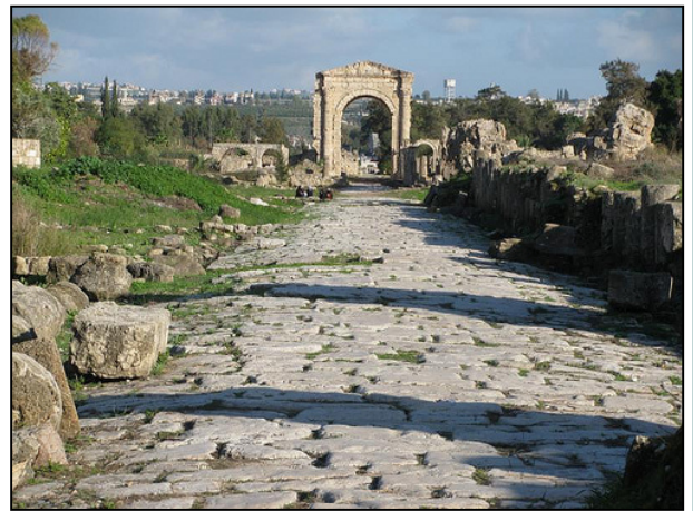
The Appian Way is crowned in middle for storm water flow.
