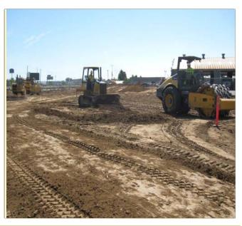
Pictured above are the building pads being graded. Some rough weather slowed this process down quite a bit since soils were saturated.
