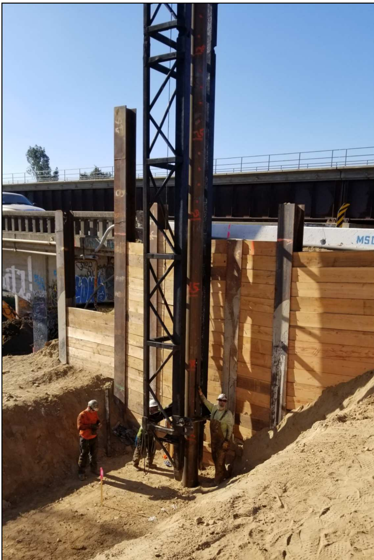
Pile driving on the north abutment
