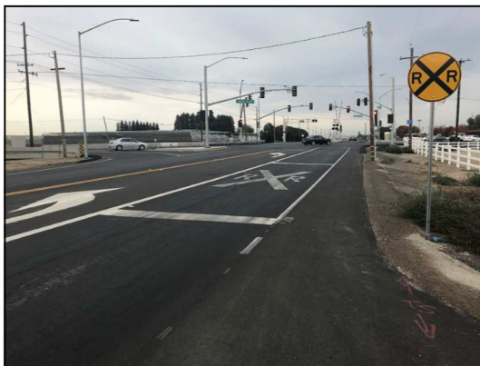
Hatch Road (Looking West) Left: BEFORE Right: AFTER
