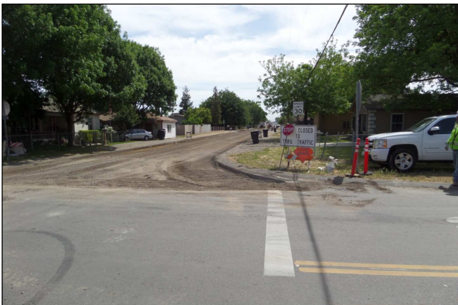
On the left—Tenaya Drive at Kerr Avenue Under Construction
