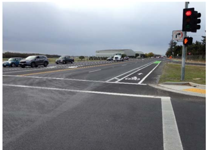
View of new asphalt rubber pavement, bike lanes and ADA accessible ramp
