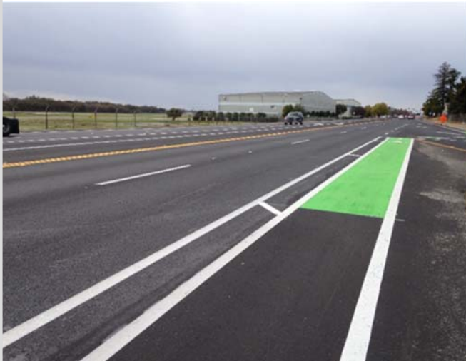
View of new asphalt rubber pavement, bike lanes and ADA accessible ramp
