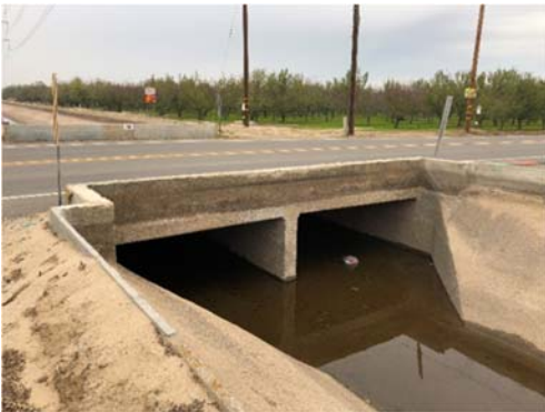
Existing view of Keyes Road at TID Ceres Main Canal
