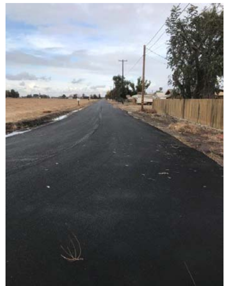
Various tree removals and road maintenance.
