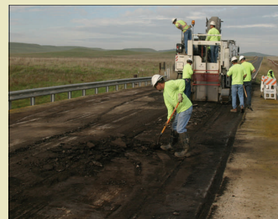
Road crews grinding asphaltic concrete off the deck.
