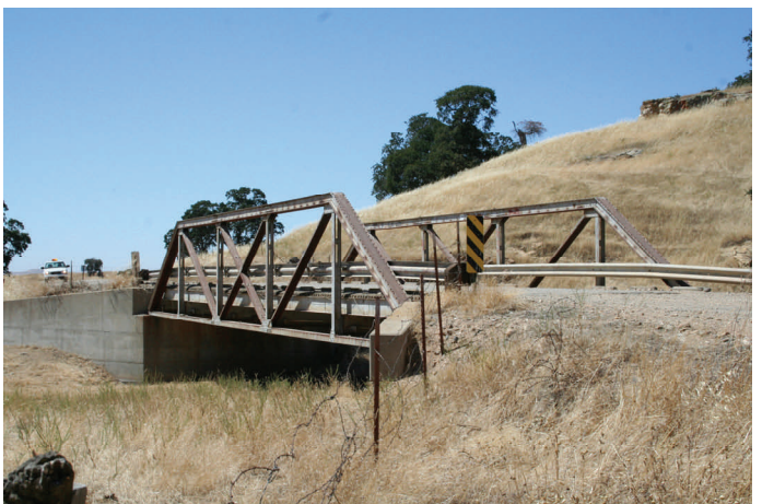
Cooperstown Road over Gallup Creek — Weight restricted Pratt Pony Truss bridge.
