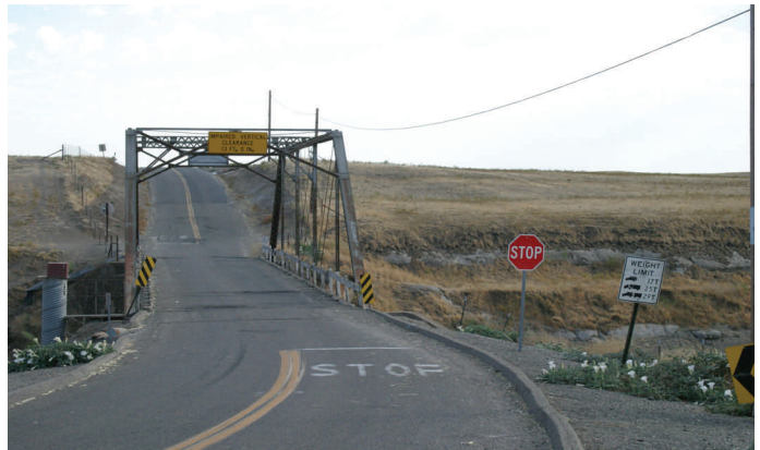
Crabtree Bridge over Dry Creek — Note the stop signs and the weight limits. The stop signs are for trying to slow down truck loads that regularly violate the weight limit on the bridge.
