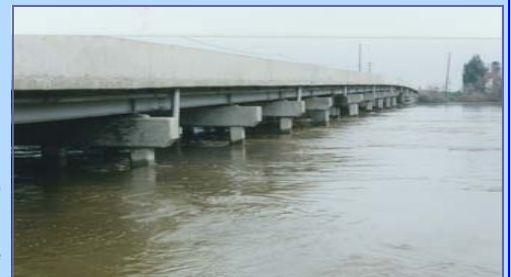
Crows Landing Road Bridge over the San Joaquin River during the 1997 Flood
