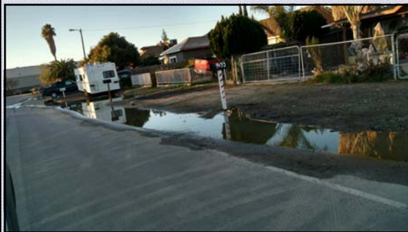
Swales filled in caused street flooding. (Photos on left and below).
