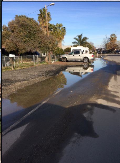
Swales filled in caused street flooding. (Photos on left and below).
