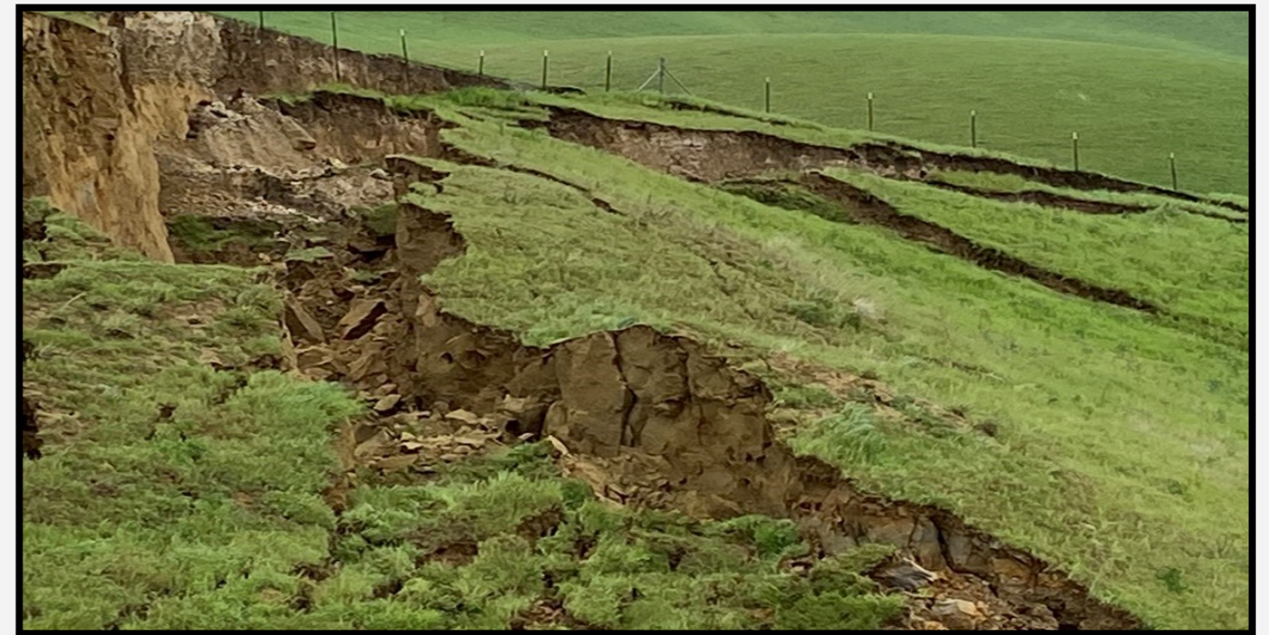
These are photos on Diablo Grande Parkway February 2023. This area is 70' high and 250' across. The whole hillside gave way due to the amount of rain that saturated the hillside. (Above)
