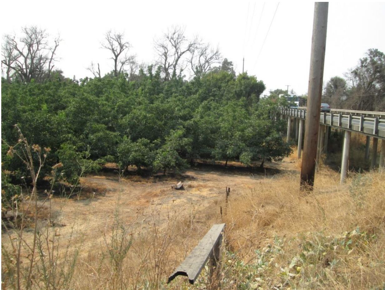
Figure 5. West side of McHenry Avenue Bridge over Dry Slough facing North.
