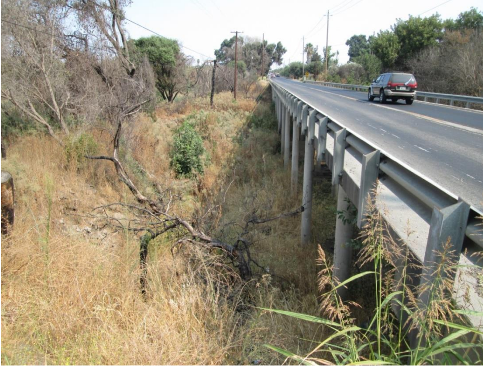
Figure 6. East side of McHenry Avenue Bridge over Dry Slough facing South.
