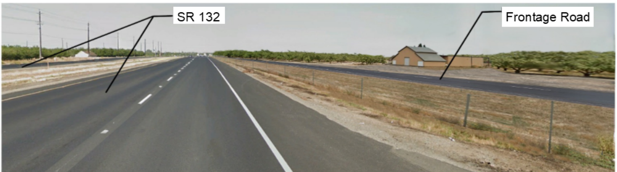
Typical frontage road adjacent to State Route 132 for Alternative 3 Looking West.
