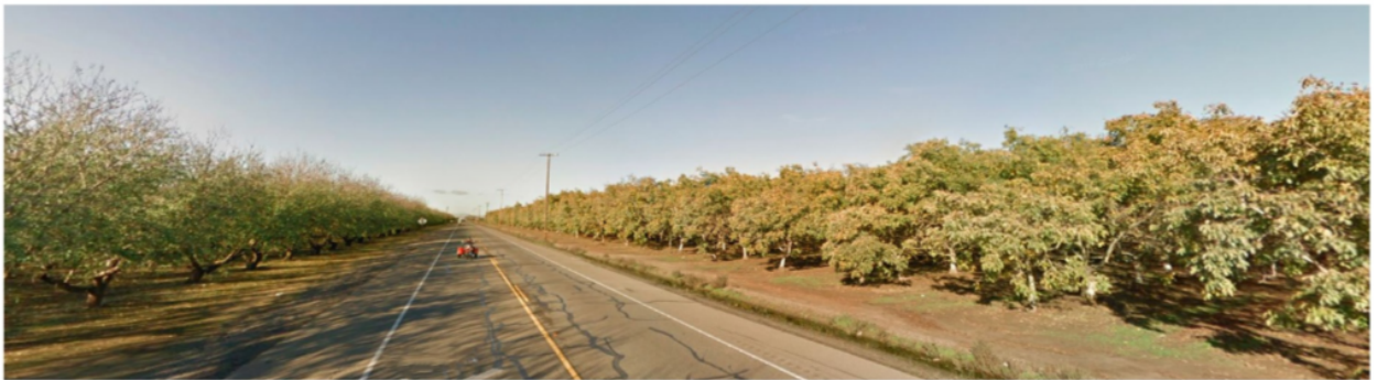
Existing condition State Route 132 looking west.
